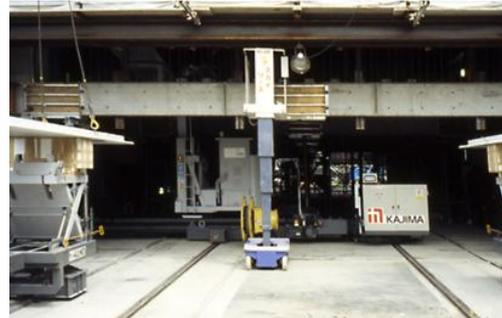
Figure 2b: Field factory with rail guided stationary production of high-rise, Kajima's AMURAD
