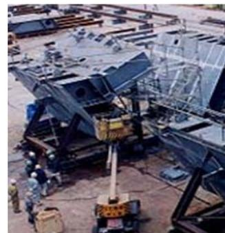
*Figure 5a, 5b, 5c: Innovation by Overlay (IbO) of new processes on existing structures: Shimizu subcontracted the production of the complex structure of the Pier to a ship yard.*
